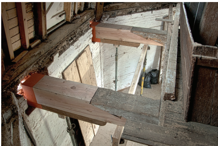
8. Scarfed ends of the sheer beams that support the Meal Floor
