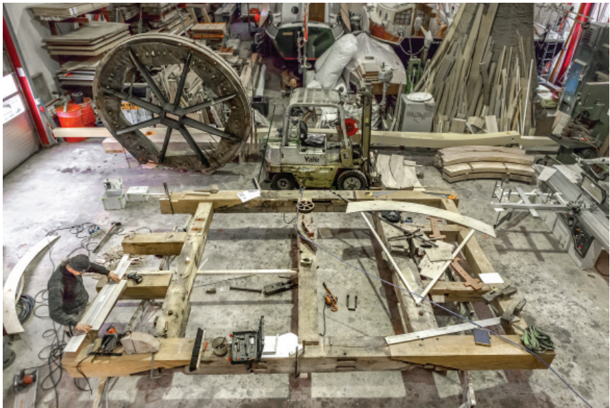
1. Cap frame during repair.
