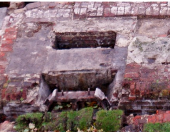
Engine plinth, and crankshaft pits
