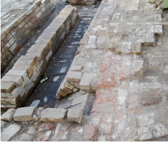
External Exhaust Flue to Chimney
