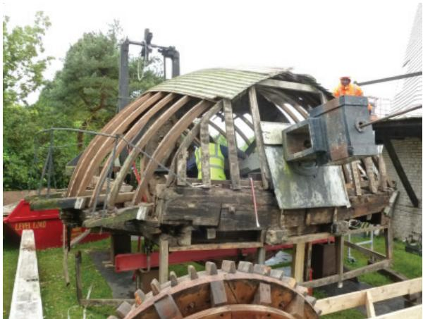
The second major lift of the day involved the removal of the upper section of the Mill's central drive shaft, complete with the wallower attached. This wooden gear wheel, its compass-arm design now rare in this country, is complete but in poor condition. It requires re-cogging and substantial repair if the Mill is to work again.
